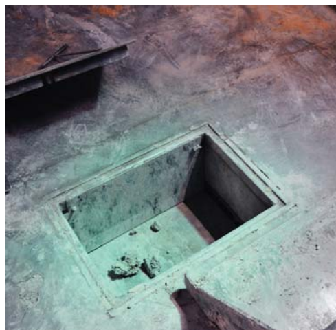
Closeable floor opening with the dimensions 60 cm x 40 cm for material drop.
