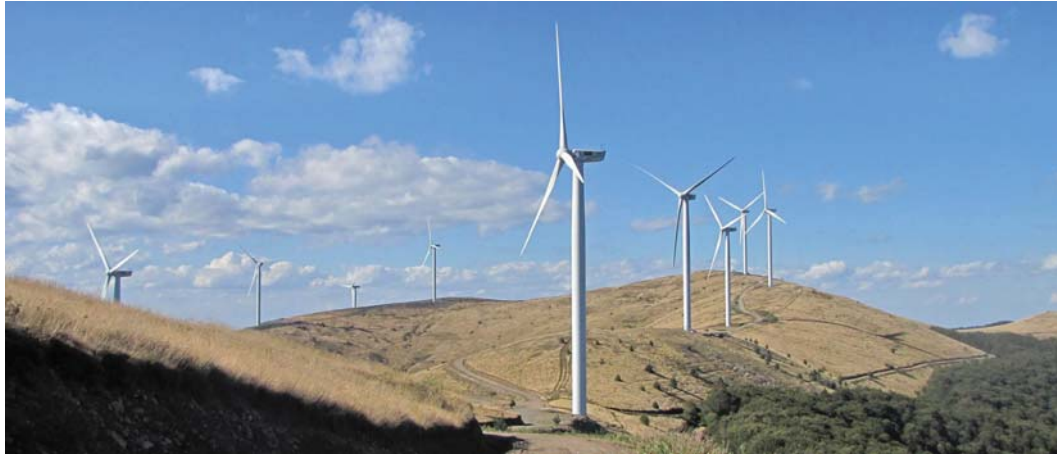
Wind park with 25 turbines of the type W2E-2.5/100 in Kazanlak (Bulgaria)
